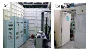
Fig. 3 (a) Fireproof wall and control panel installed in nonexplosion-proof area and (b) protective wall isolating the individual testing devices
