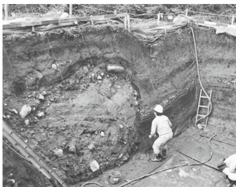
Fig. 1 Example of trench investigation of an active fault (Nukumi Fault of the Nobi Fault zone, Ohno City, Fukui Prefecture).
