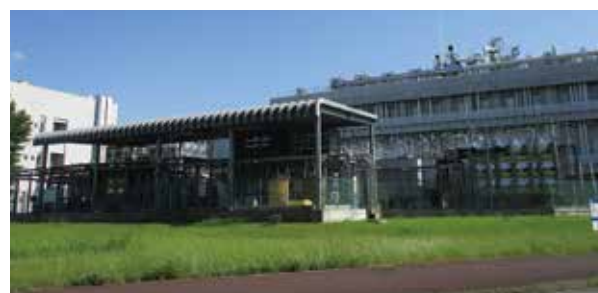
Wastewater treatment plant at AIST Tsukuba
