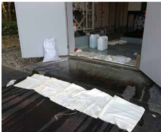
Emergency accident drill supposing light oil* had leaked while refueling in the room for a house power generator for emergency and flowed outside (*water used for the drill)
