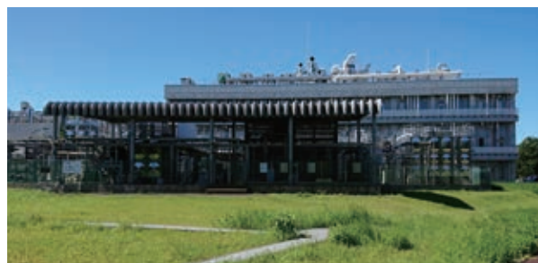
Wastewater treatment plant at AIST Tsukuba
