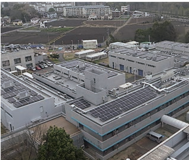
Tsukuba West building group 4 equipped for energy efficiency including building West 4A, which attained 5* ZEB, with 179 kW capacity of solar panels on the roofs (equivalent to that of 35 ordinary houses)
