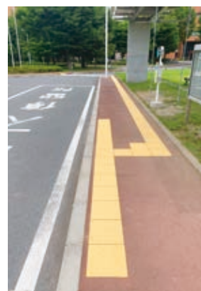
Installing tactile paving
