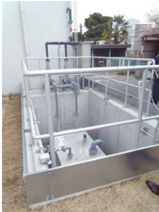
Tank pit with a raised wall
