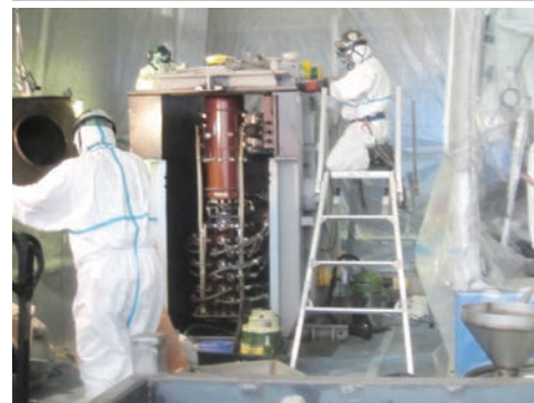
A transformer being disassembled
