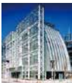
AIST Tokyo Waterfront Main Bldg.
