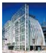
AIST Tokyo Waterfront Main Bldg.
