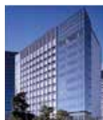
AIST Tokyo Waterfront Annex (Bio-IT Research Bldg.)
