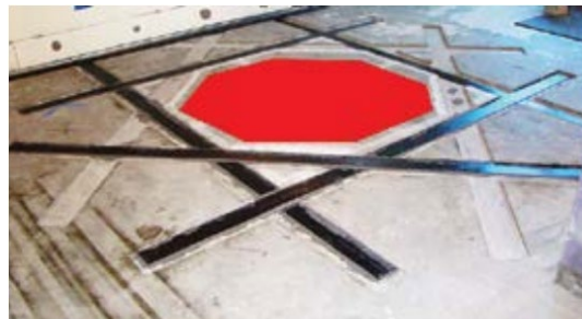
Fig. 10: Octagonal cut-out in slab reinforced with CFRP laminates
