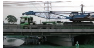
Monitoring a bridge in use
