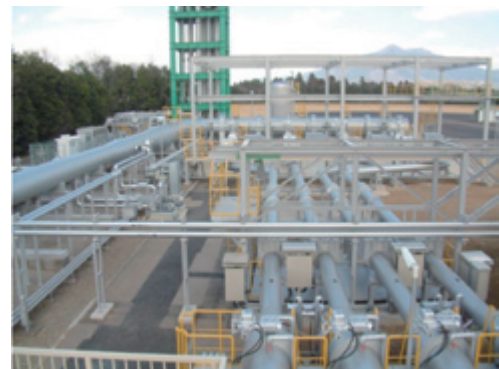
Figure 2: Hot water circulating channels and working standard flowmeters.
