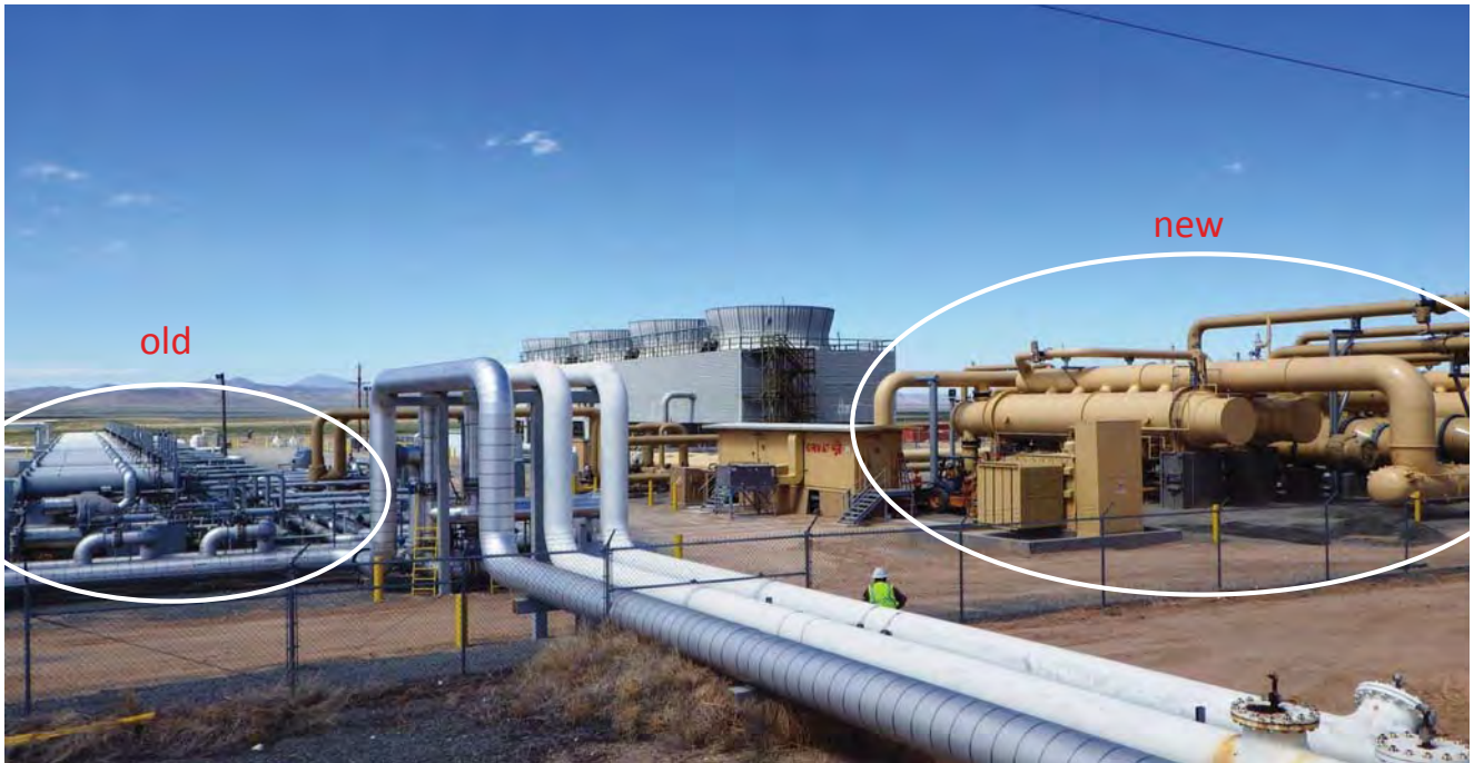
New Project: Cove Fort, Utah
