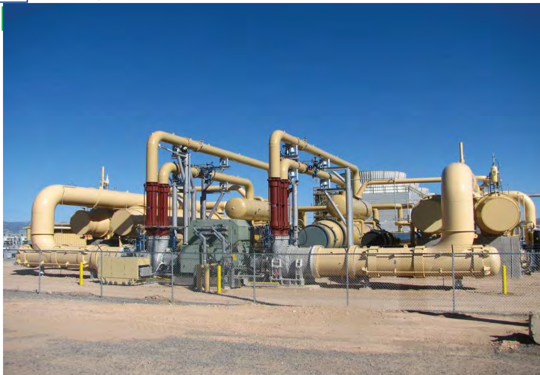
New Project: Cove Fort, Utah
