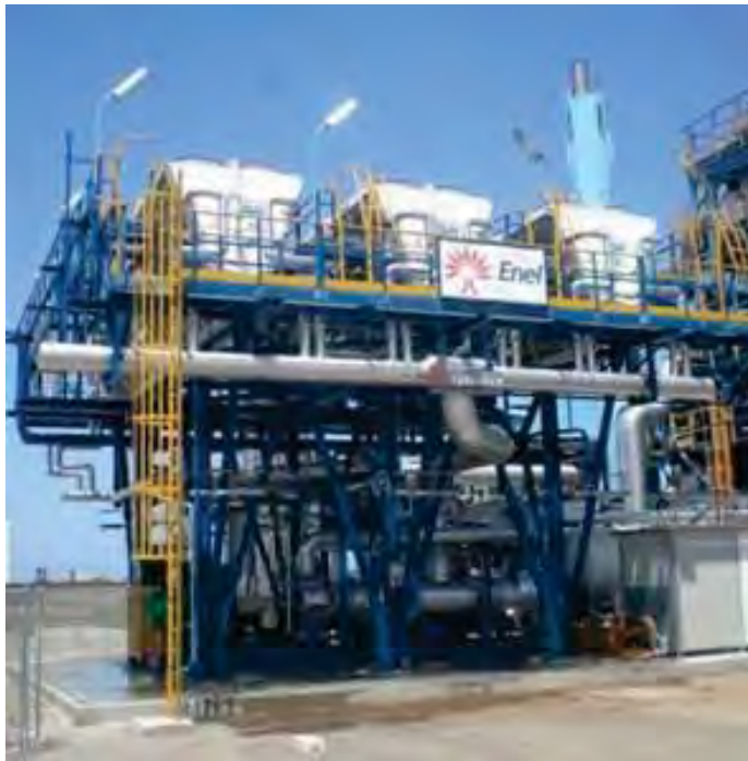
Experimental campaign – ORC power plant prototype realization
