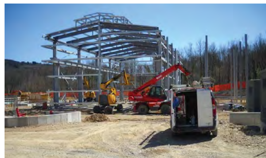
Building machinery erection
