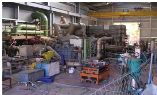
Main machinery erection
