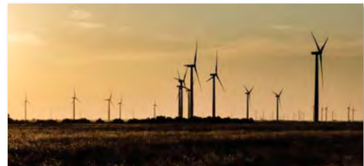
Projects in execution
