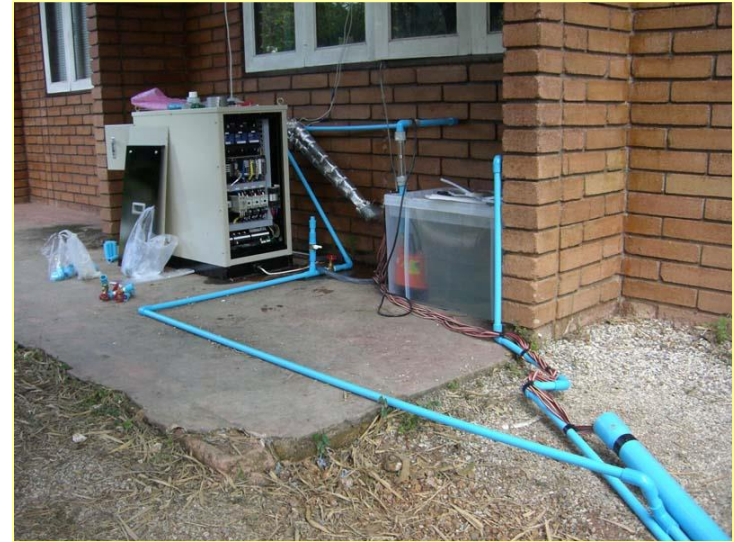
GHP and Water Circulation System
