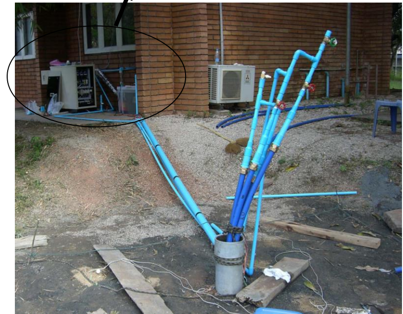
Double U-tubing in 56m Depth Well.
