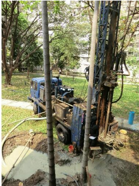
Drilling for 50m
