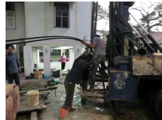
PE Pipe Setting to 50m Depth (100m length)
