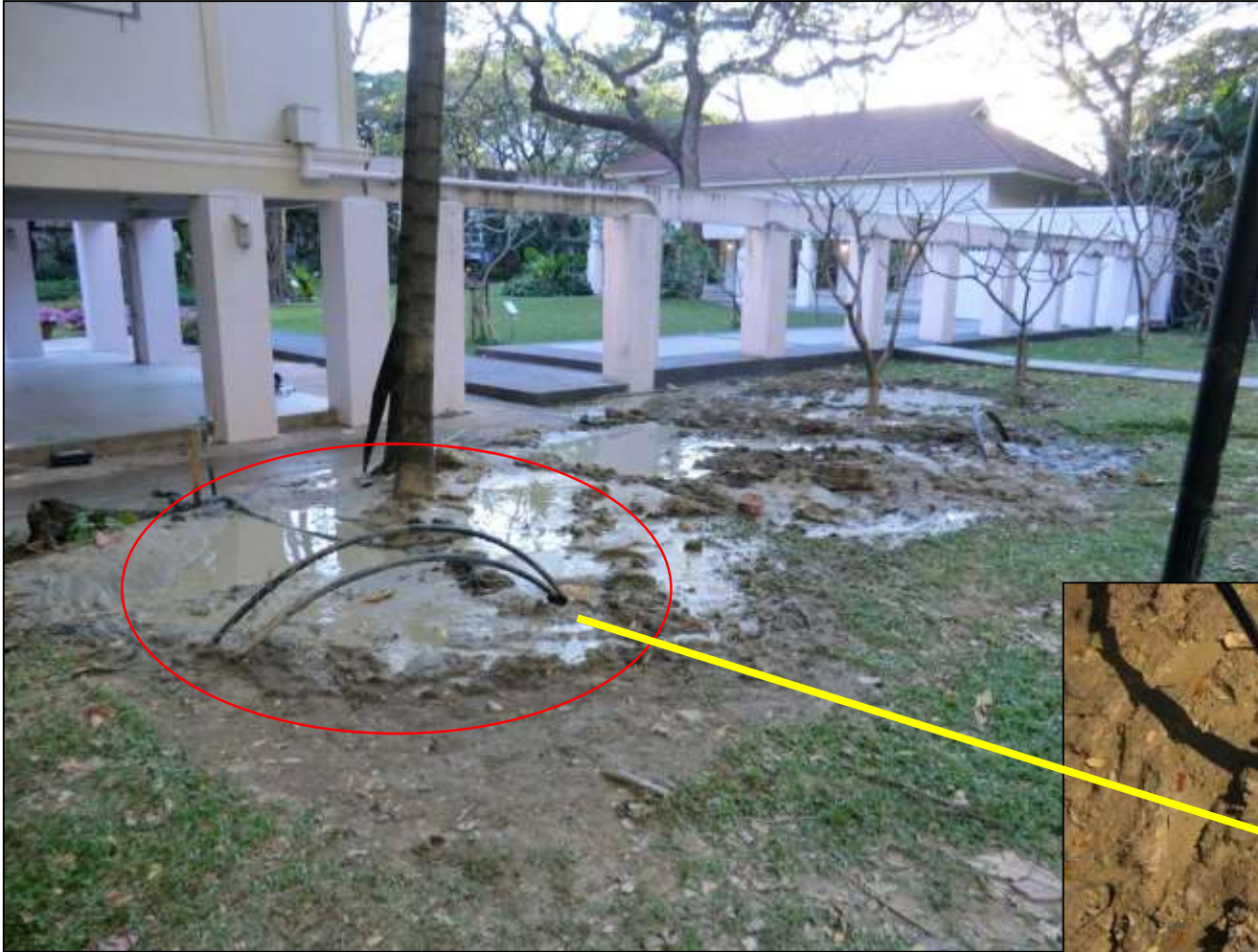
After installation of heat exchange pipe
