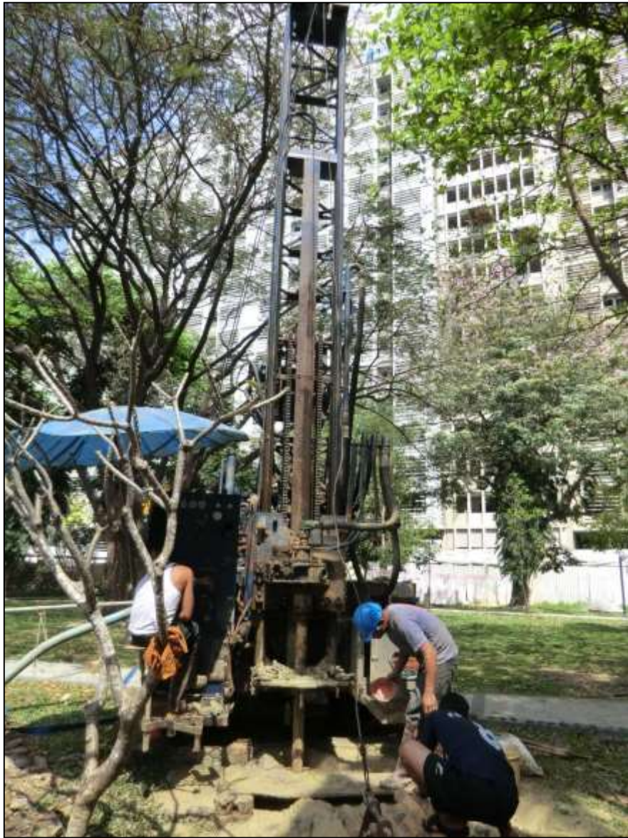
Drilling for installation of heat exchanger
