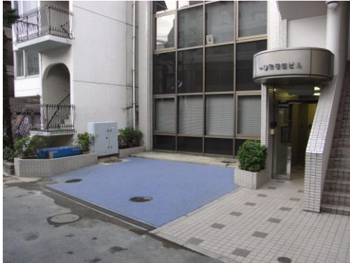
Parking Lot where 8 ground heat exchangers of 75 m in length are settled
