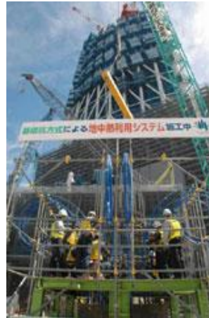
Ground heat exchanger under construction (Taisei Corporation)
