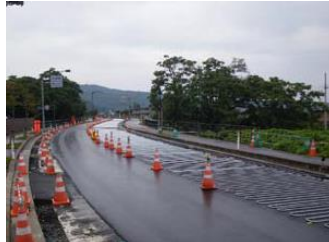
Snow melting system under construction (JGD)
