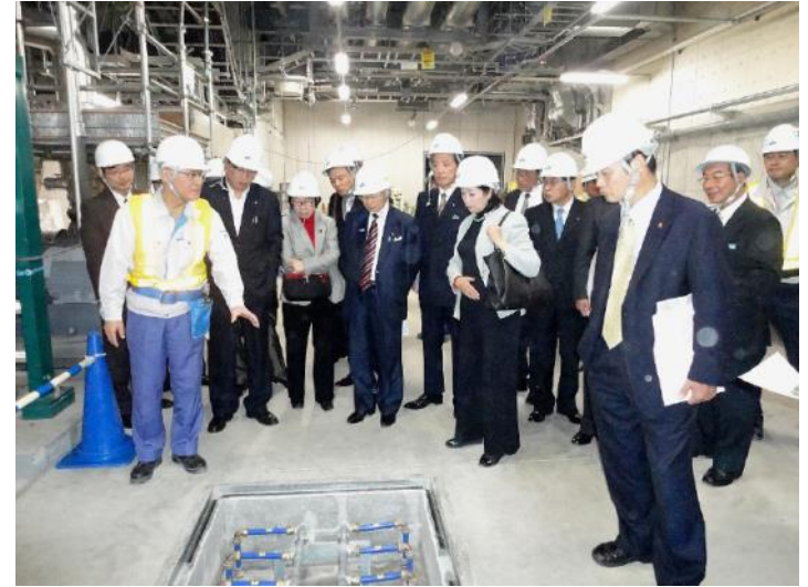
Ground source heat pump system and the Diet Members
